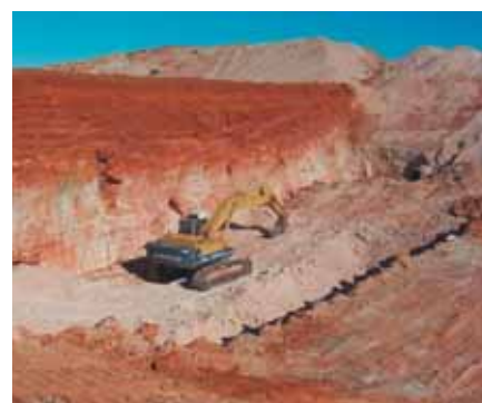
Trench digger in a bulldozer cut. (Photo 049377)
