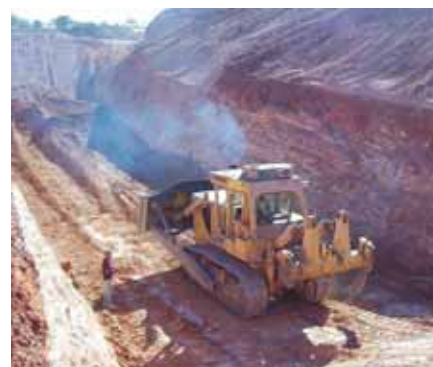
Bulldozer in an open cut. (Photo 049378)
